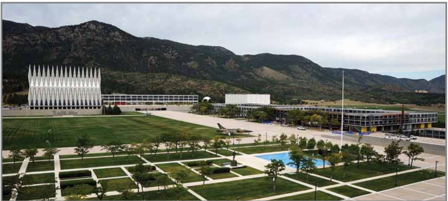
Above: The Air Force Academy's Cadet Chapel, designed by Walter A. Netsch, Jr., is the most popular man-made attraction in Colorado, with more than a half million visitors every year. Construction on the aluminum, glass and steel structure began in 1959 and was completed in 1963 at a cost of $3.5M; Vandenberg Hall, at right, houses more than 2,000 cadets and is undergoing a multi-phase, multi-year renovation. Upper right: USAFA is home to several world championship Firefighter Combat Challenge teams, including the competitors shown here participating in "Rumble in the Rockies," a regional event with 40 teams participating at Falcon Stadium on the Academy. (U.S. Air Force photos)
