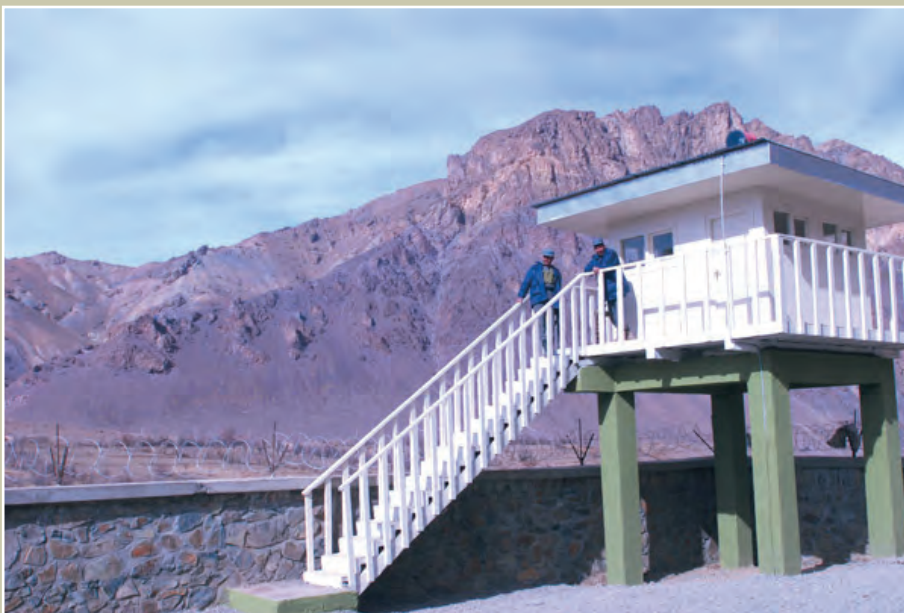
Two Afghan National Police (ANP) soldiers occupy a guard tower recently completed by the Corps of Engineers to provide lookout over the Surkhi Parsa Valley in Parwan Province. (U.S. Army photo)
