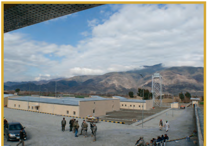
The Afghan Border Police Station, a U.S. Army Corps of Engineers project, was built by Afghan contractors. (Photo by TSgt Jason Jenkins)
