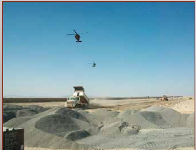
RED HORSE Airmen spread-dump and grade base course across the runway.
