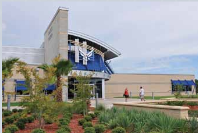
The new Tyndall Fitness Center is the first Air Force facility to achieve the U.S. Green Building Council’s LEED Platinum rating. (photo by Ms. Lisa Norman)
