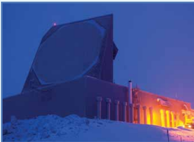
One of the two radar faces of the Ballistic Missile Early Warning System, or BMEWS, site is shown during a short period of twilight at Thule AB, Greenland. (photo by Mr. Michael Tolzmann)
