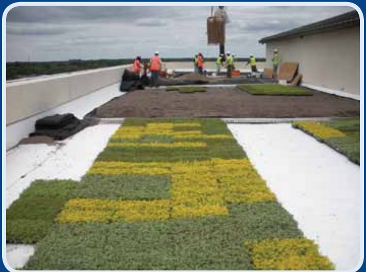
Workers plant vegetation on the rooftop of the new BRAC/ National Capital Region Relocation Administrative Facility at JB Andrews, Md. (photo by Ms. Summer Allen)
