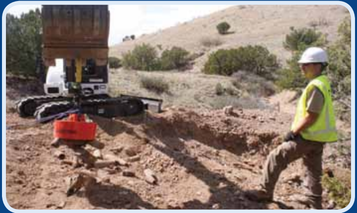
A worker uses an industrial magnet to remove munitions debris from a mine shaft at Kirtland AFB, N.M., as part of the military munitions response program. (courtesy photo)
