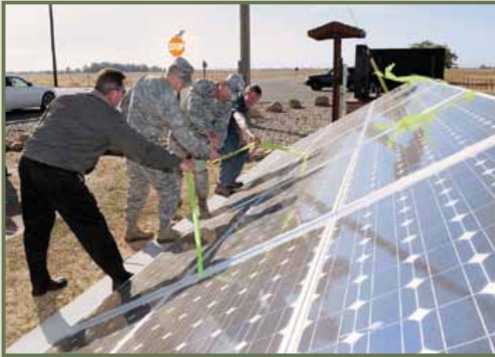
At Beale AFB, Calif., a solar array powering the base’s main gate information marquee began operation with a ceremonial ribbon cutting. (photo by Mr. John Schwab)
