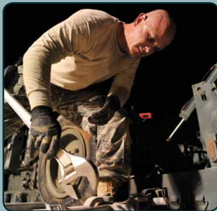
SSgt Brian Seabolt, 380 ECES, tightens a bolt on a mobile aircraft arresting system during a two-week maintenance overhaul of the system. (photo by TSgt. Patrick Mitchell)
