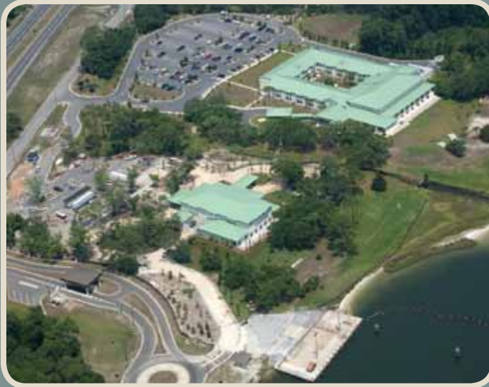
Construction of Hurlburt Field’s Joint Mission Planning Facility (foreground) and the now completed Soundside Club and Visitor’s Quarters (background)(photo courtesy of Aero Photo)
