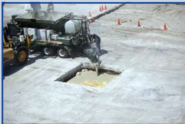
1Lt Andrew Kopeikin (top photo), AFRL researcher, with sensor-equipped T-16 UAV provided by Idaho National Laboratories. MTLs with attached rock saws (middle photo) cut away upheaval while an excavator waits to remove it. Members of 823 RHS (bottom photo) place rapid setting concrete over high density foam using a new continuous mixer. (photos courtesy of ERDC)
