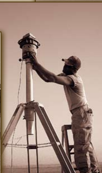
Photo left: Local Contractors deliver hundreds of loads of aggregate material by tractor, the only means available to them. Photo middle: TSgt Kendall Long tightens down the rotating laser transmitter. (photos by MSgt Gerald D. Haight) Photo above: The newly constructed airstrip at FOB Dwyer, Afghanistan, welcomes its first fixed wing aircraft, a C-130 that successfully landed on the AM-2 matting surface on Aug. 27, 2009. (photo by TSgt Robert N. Cullison)
