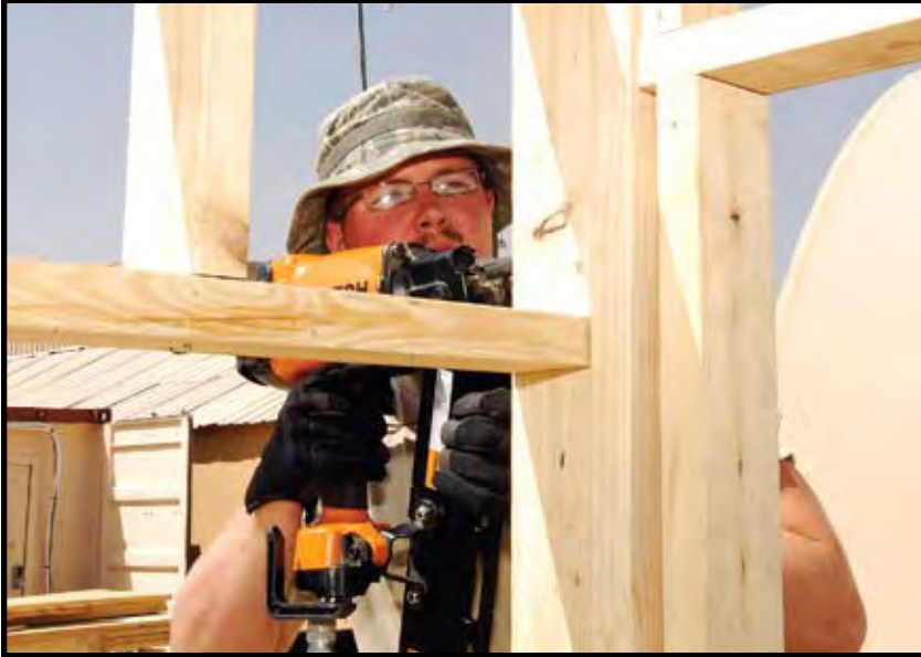
SrA Eric Horn, 455 ECES, uses a nail gun to build a flight line guard shack at Bagram Airfield, Afghanistan. (photo by SrA Felicia Juenke)
