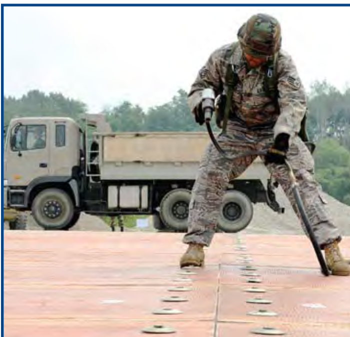
Photo left: SSgt William Deguzman uses an pneumatic drill to connect two folded fiberglass mats together on a simulated runway at Jungwon AB, Republic of Korea. (photo by SrA Stephenie Wade) Photo right: A1C Brandon Wood shovels dirt into a sand bag at Eielson AFB, Alaska. (photo by A1C Laura Goodgame)
