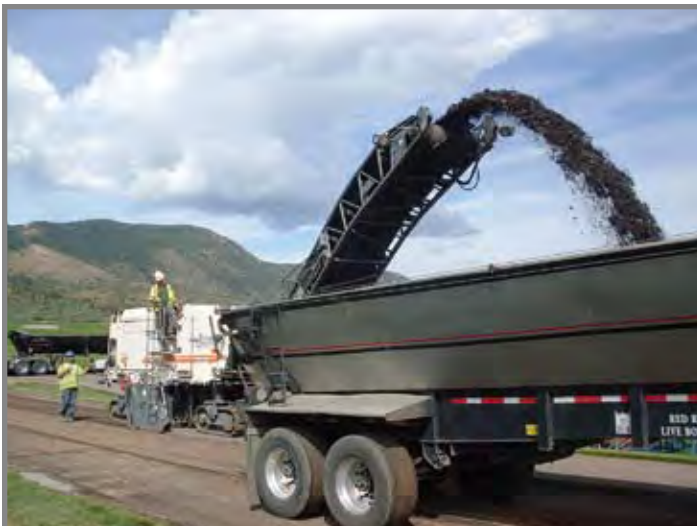
Photo Below: Contractors mill a section of South Gate Boulevard, part of a $3.5M full-depth repair of 10 lane-miles of the Academy’s main thoroughfare. Photo Right: Firefighter Ron Prettyman competes in a regional Scott Firefighter Combat Challenge hosted by USAFA. (U. S. Air Force photos)
