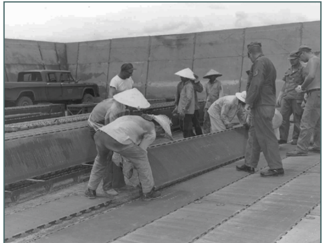
Prime BEEF engineers and local laborers lay AM-2 in a protective revetment at Tan Son Nhut AB, Vietnam. (U.S. Air Force photo)
