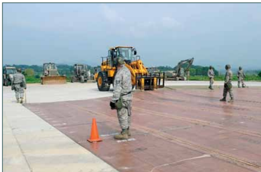
(below right) An engineer tightens the bolts to anchor the fiberglass mats in place. (U.S. Air Force photos)
