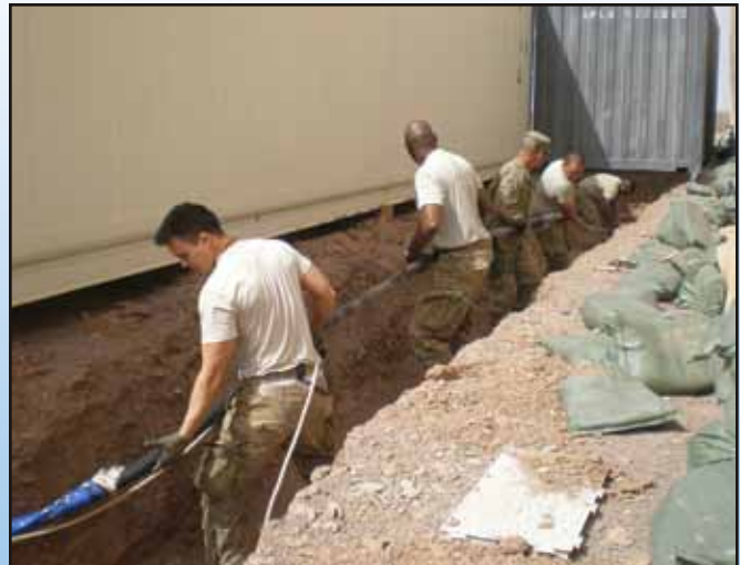
(above and below) Members of the 577 EPBS and Shindand AB’s troop labor volunteers install electrical cable to supply power to the base’s dining facility in Afghanistan. (U.S. Air Force photo)
