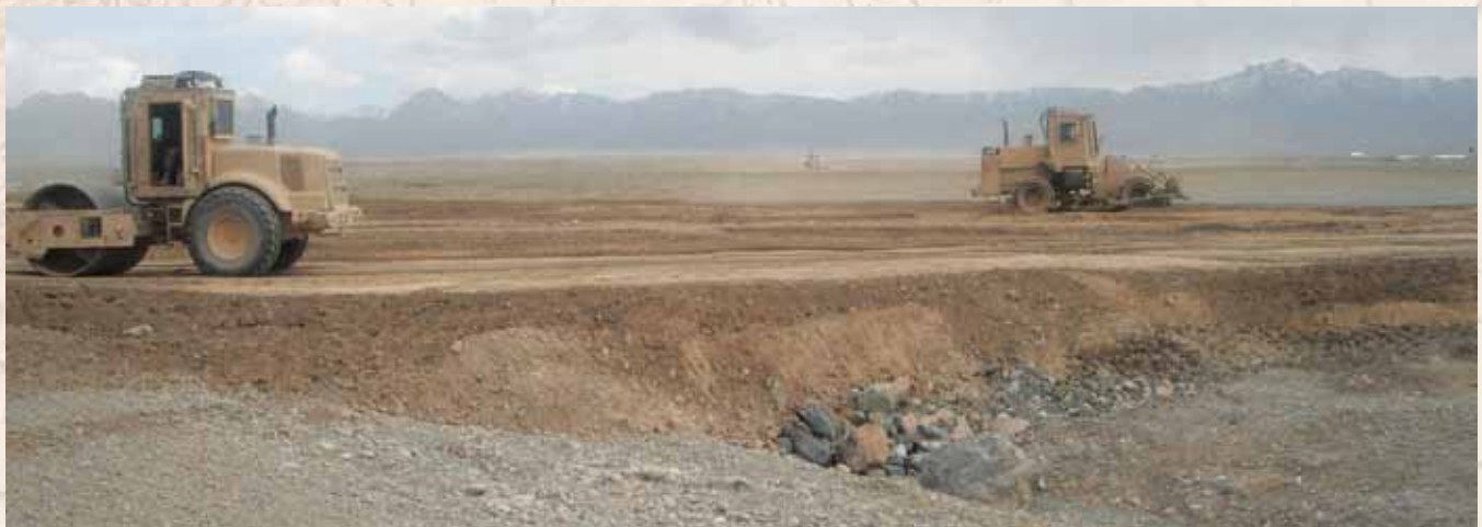
(below) The final compaction pass — the land bridge is at final grade. (photo by Mr. E. John Schumacher)
