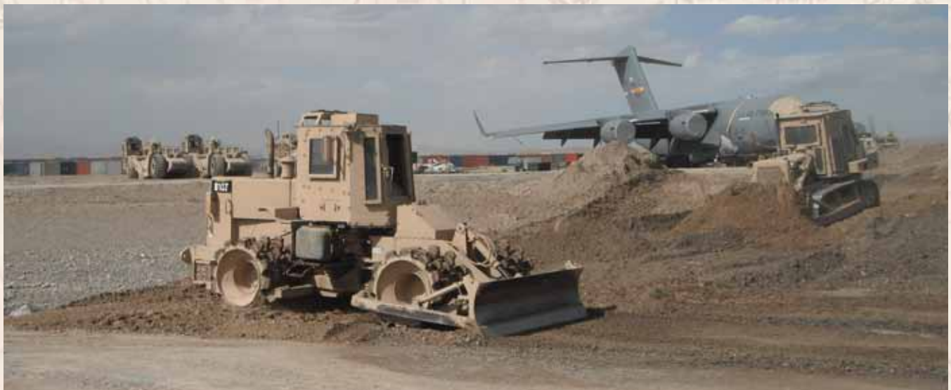
TSgt Livingston and SSgt Resendez place side slopes over coarse aggregate. (photo by Maj Mel Ibarreta)
