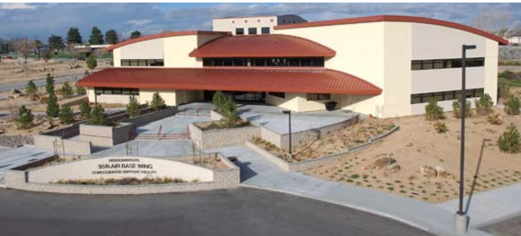
The Edwards AFB Consolidated Support Facility earned LEED Silver certification. (U.S. Air Force photo)
