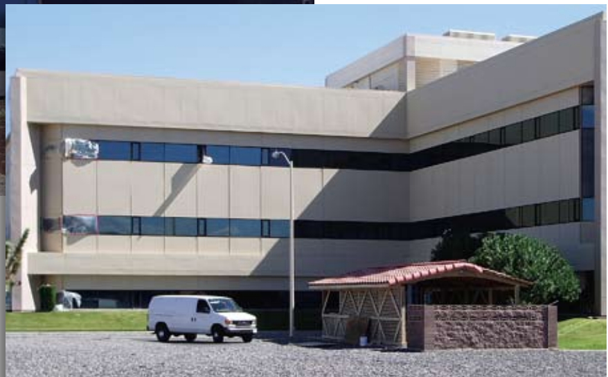
Glass spandrels (above) on Nellis AFB's Consolidated Support Facility "helped" raise the cooling load. Painting them over with a special ceramic coating (right) reduced the load and cooling costs. (U.S. Air Force photos)
