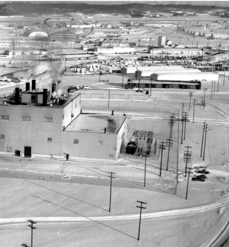
AFB's half-century-old co-generation plant was replaced by switching to the local system exceeded the guaranteed consumption savings by 27%.
