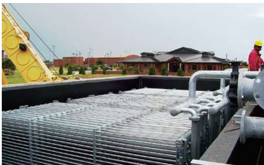
Built using an ESPC, Dyess AFB's ice plant cools 13 buildings on the Texas base by distributing water cooled by ice produced at night, when the temperatures are at their lowest. (U.S. Air Force photo)
