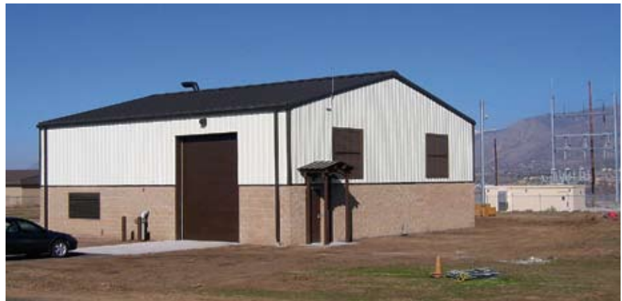
Landfill gas-to-energy plant at Hill AFB (U.S. Air Force photo)
