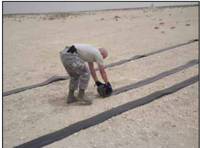
Following removal of the aircraft arresting system barriers, SMSgt Stephen Burns rolls the worn nylon tape that will be replaced as a part of the overhaul process. (U.S. Air Force photo)
