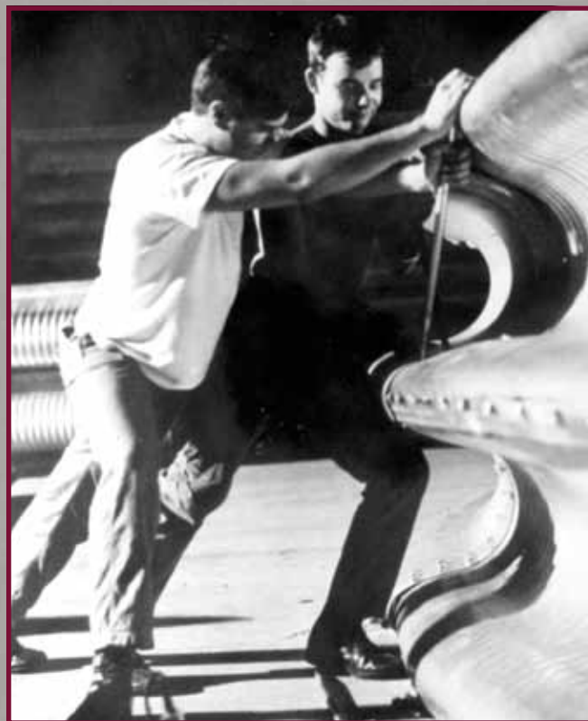
Working projects outside their career field specialty areas was a way of life for many. Electricians and plumbers operated paving trains and all craftsmen helped erect aircraft revetments. (courtesy photo)
