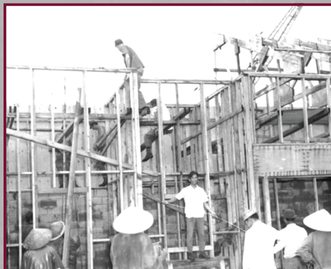
(below) A 4,800-squarefoot operations building, completed in just 31 days thanks to pre-fabricated wall and roof components and a fast-tracked schedule. (courtesy photo)
