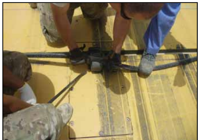
The team reattaches the arresting cable to one of the rubber support blocks on one of the BAK-14 systems. (photo by SMSgt Stephen Burns)
