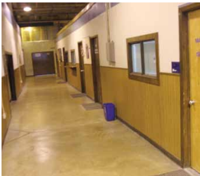
A FOCUS project at JB San Antonio-Lackland, Texas, renovated the 433rd Airlift Wing Headquarters exterior and interior, shown before the project (above) and after (below). (U.S. Air Force photos)
