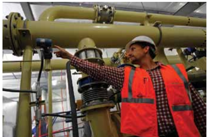
Mr. Greg Mitchell, JBER's LFG power generation facility operator, checks the pressure on a gas processing module. (photo by TSgt Brian Ferguson)
