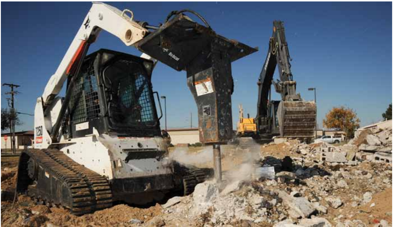
A member of the 22 CES horizontal shop uses a skid steer loader with a hammer attachment to demolish a building on McConnell AFB, Kan. (photo by A1C Jose L. Leon)
