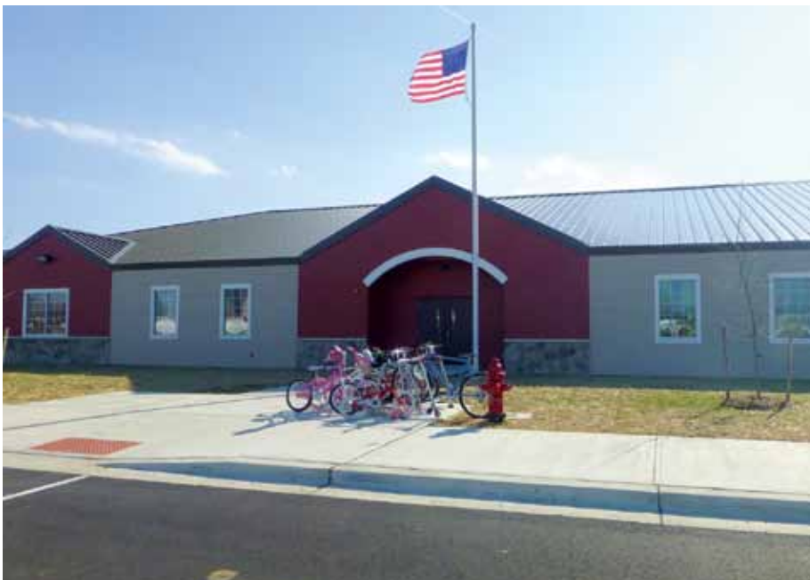
Front entrance of the Imagine Andrews public charter school located on Joint Base Andrews-Naval Facility Washington, Md. (U.S. Air Force photo/DeAnne Edlund)
