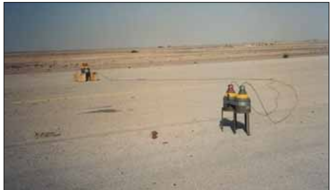
(below) Shaped charges were used to blow the initial holes in the runway which would then be expanded using other munitions. (U.S. Air Force photo)
