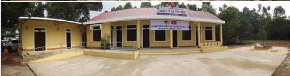
Before and after photos of the medical clinic at Dong Hoi, Vietnam, following renovation by an 18-person U.S. military engineering team that included Air Force CEs. (courtesy photos)
