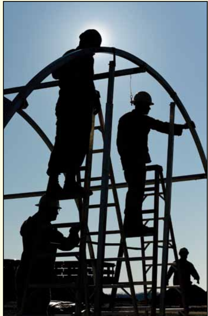
Prime BEEF Airmen from the 436th Civil Engineer Squadron assemble a tent frame during a training deployment to Dover AFB, Del. (U.S. Air Force photo/Roland Balik)
