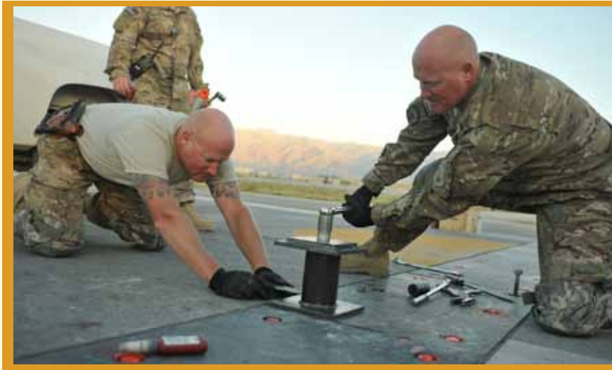
Master Sgt. Joshua Graves (left) and Master Sgt. Jeremiah Graves, brothers deployed from the Guard's 148 Civil Engineer Squadron, work on runway repairs at Bagram Field, Afghanistan. (U.S. Air Force photo/Airman 1st Class Bobby Cummings)
