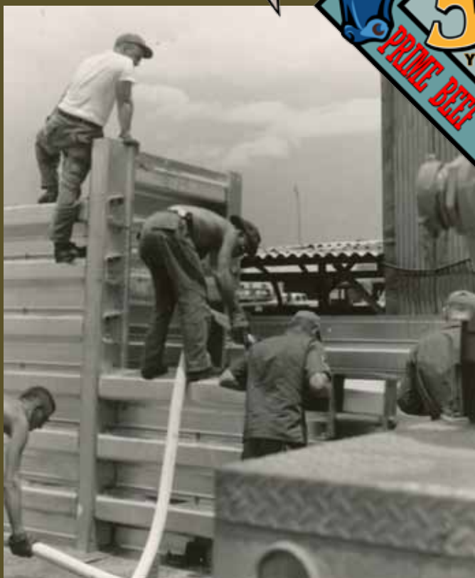
Members of Prime BEEF Team I construct revetment at Tan Son Nhut AB, Vietnam, in 1965.
