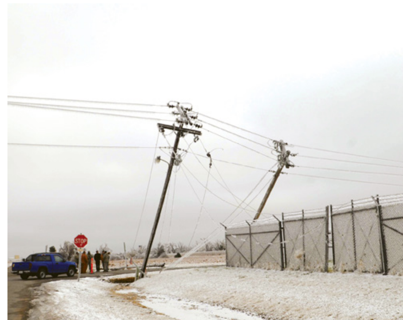
97th Air Mobility Wing emergency management personnel talk with Dan Scott of the City of Altus and Mike Hagy of Southwest Rural Electric to discuss the downed power lines outside the Jasmine gate at Altus Air Force Base, Oklahoma, on Jan. 30, 2010. A devastating ice storm that hit Jan. 28 left more than 30,000 people without power in the Altus area. (U.S. Air Force photo by Senior Airman Leandra D. Hernandez)
