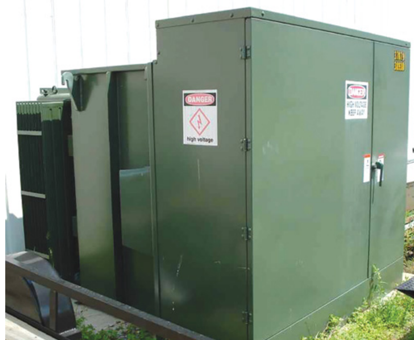
ABOVE: A pad-mounted transformer is a ground-mounted electric power distribution transformer in a locked steel cabinet mounted on a concrete pad. LEFT: Steel poles last 10 years longer than wooden ones. (Courtesy photos)
