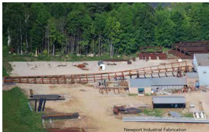
▲ Pre-assembly work in the fabrication shop yard.
