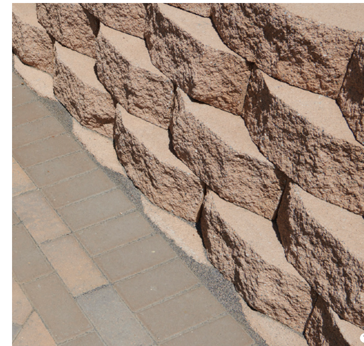
1. Tan 16" Planter Wall in a common bond pattern. Pavers are Courtyard Stone in Tuscan installed in a 45 degree random ashlar pattern. Border is Holland Mocha soldier course, Holland Tuscan in a running bond and Holland Mocha in a running bond.
