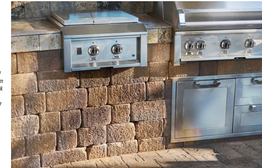
1. Sand-Stone-Mocha Stonewall® II block and cap planter wall. Pavers are Courtyard Combo Sand-Stone-Mocha installed in a random ashlar pattern. Border detail is Holland Mocha in a soldier course, with running bonds of Holland Sand-Stone-Mocha and Holland Mocha. 2. Tuscan Stonewall® II block installed in a BBQ in a random ashlar pattern. 3. Tuscan Stonewall® II block and cap installed in a random ashlar pattern. Pavers are Estate Cobble I & II (tumbled) in Tuscan installed in a random ashlar pattern. Border is Estate Cobble II (tumbled) in solid Mocha (special order). 4. BBQ is Tuscan Stonewall® II block and cap custom built onsite by the contractor. Pavers are Slate Stone in Dark Gray-Copper-Charcoal (special order) installed in a random ashlar pattern. Banding is Slate 6x9 in solid Charcoal. Circle is Slate Circle in Gray-Charcoal.
