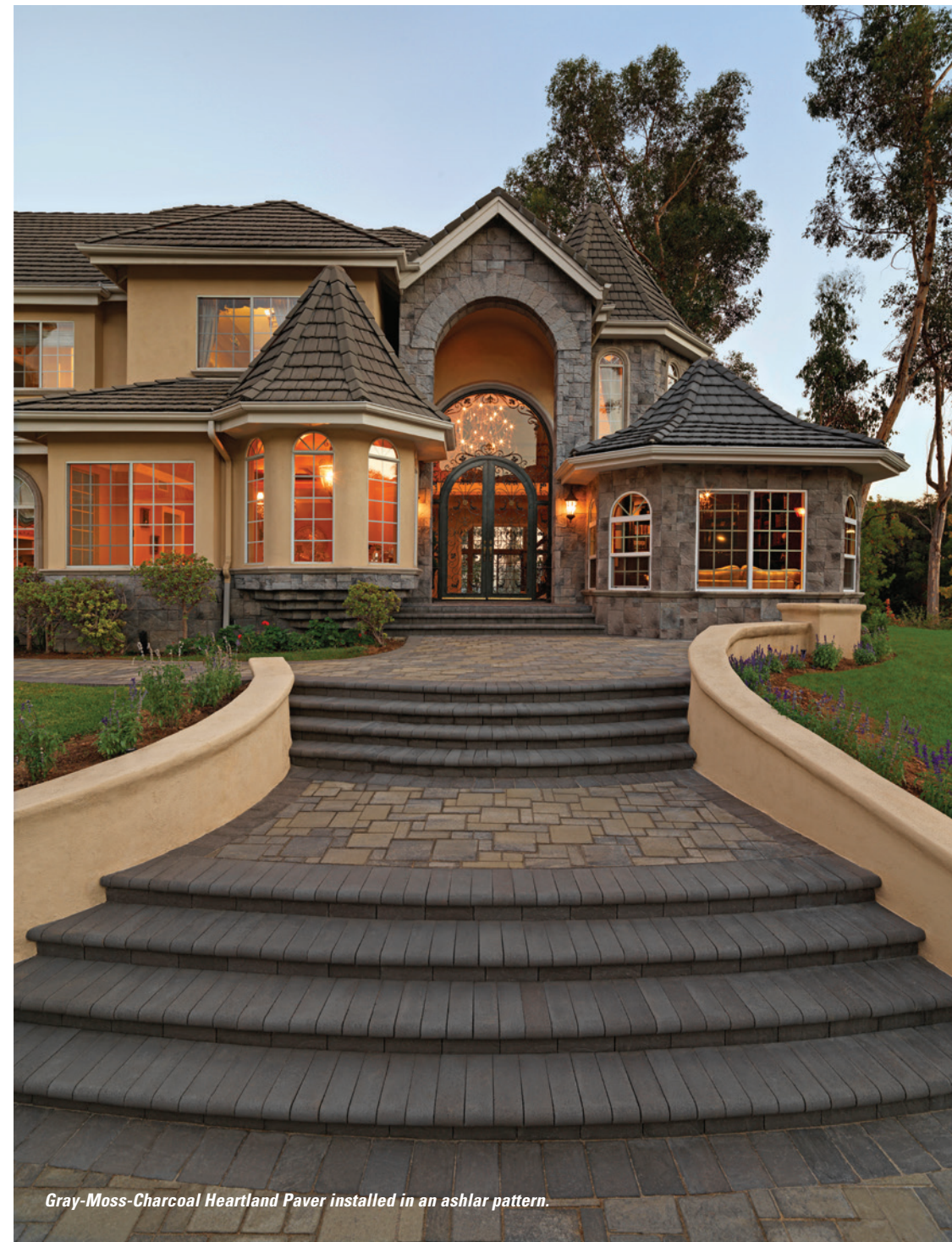
Gray-Moss-Charcoal Heartland Paver installed in a random ashlar pattern. Border is 6x12 Gray-Charcoal installed in a soldier course (note: 6x12 is a special order item).
