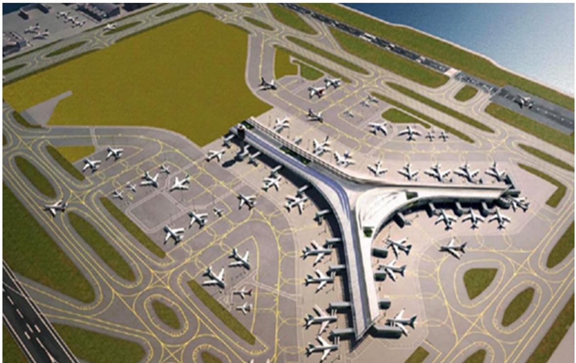
圖 28 Third Runway Concourse Phase 1 2023
