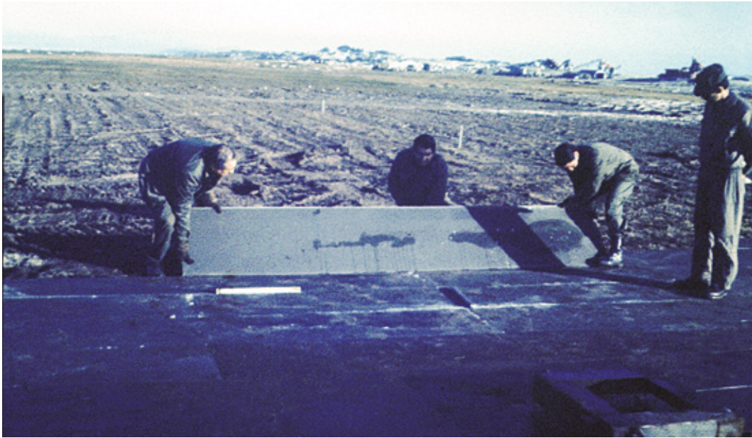
Installation of aluminum plates at BAM Malvinas - Photo courtesy of: Com. VGM (R) Grünert
