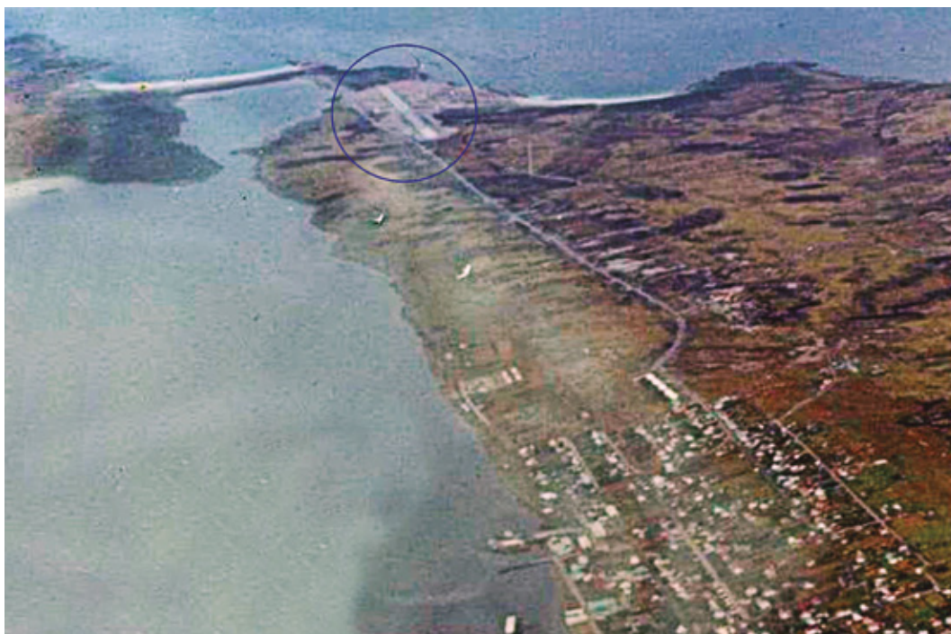
The aluminium airstrip, build by Grupo 1 de Construcciones at Hookers Point, 2 km Stanley Port
