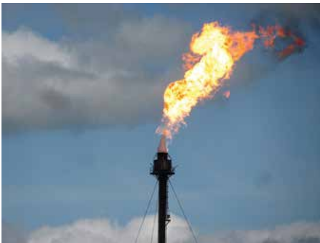
Petrochemical plants use flaring to consume waste gases by combusting them in an open flame.
