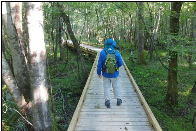
Hiker crosses long boardwalk bridge over Canady Branch.
