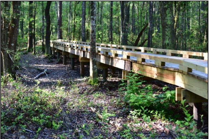
Many boardwalk bridges keep you dry from the swamp habitat.
