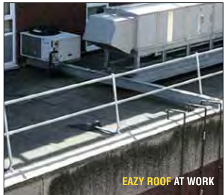
EAZY ROOF AT WORK
