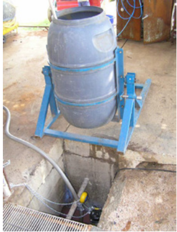
Figure 13. Tipping drum in position beside sump.
