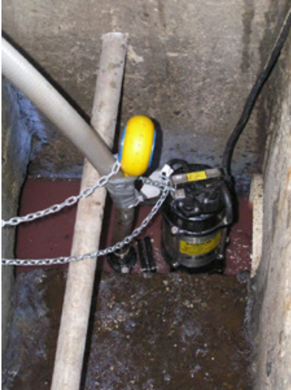
Figure 12. Davey D120GA submersible grinder pump installed in sump for collection of shed effluent samples.
