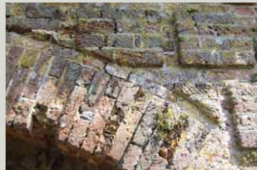
Rusticated brickwork at Ballyannan, Co. Cork. The detailed view shows beautiful axed work
