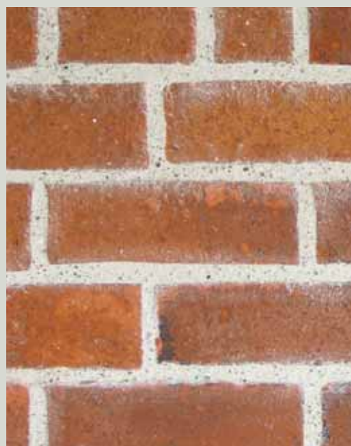
Recent repointing of a brick wall with a lime-based mortar
