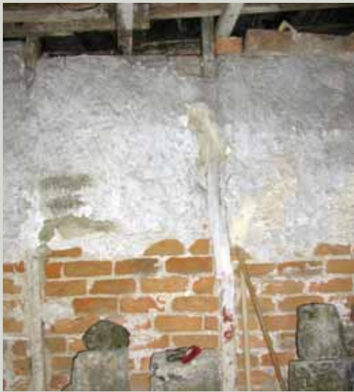
Handmade brick used in a brick nogged internal partition, now exposed where the original plaster coating has fallen away
