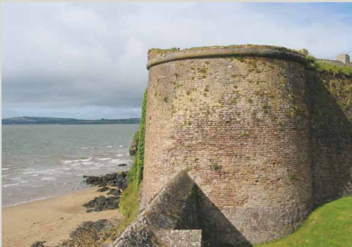
Duncannon Fort, Co. Wexford was partly repaired and rebuilt in Flemish bond brickwork during the eighteenth century
