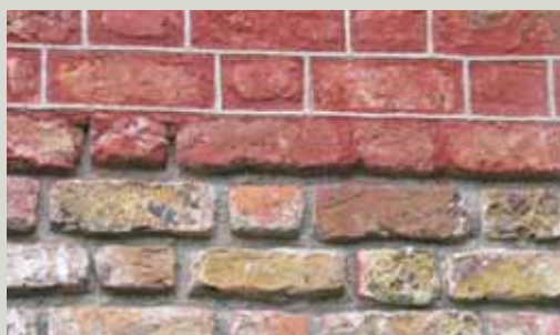
Tuck pointing in practice
