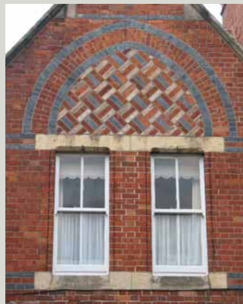
Polychromatic brickwork at the Mageogh Home, Rathmines, Dublin dating from 1878
