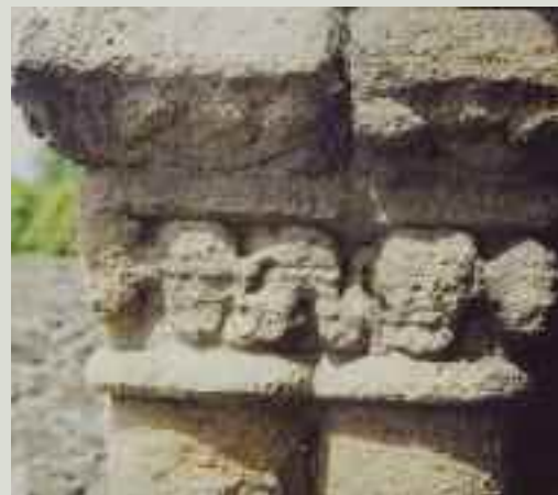
Carved sandstone, showing weathering. Sandstone was widely used for carving because it was relatively soft and easily worked. Some high crosses and Romanesque detailing were carved in sandstone
