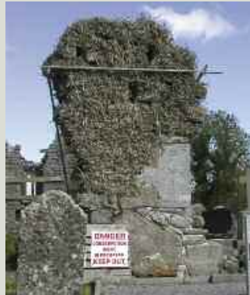
A clear sign warns of conservation works in progress. The temporary works to the wall in the background include scaffolding poles to provide restraint. The concrete blockwork on the right hand side provides temporary propping pending reinstatement of the wall core
