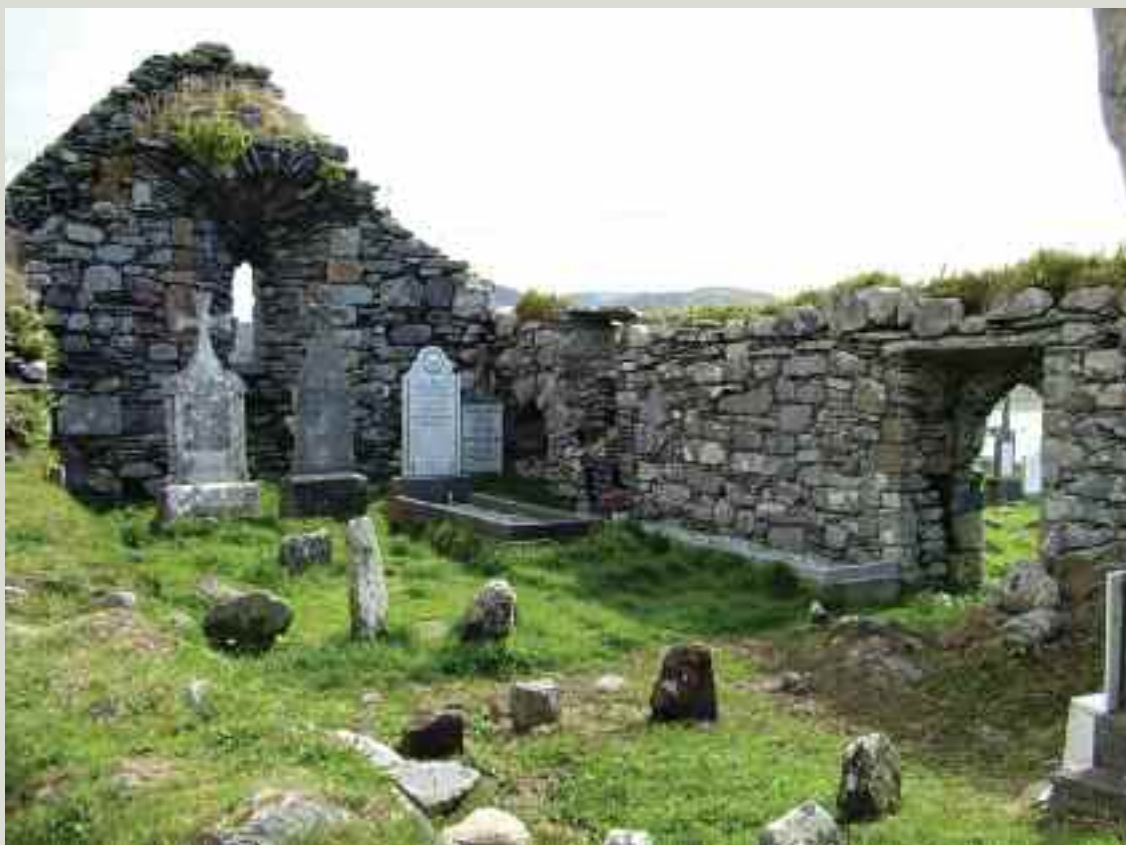
Graves close to a ruined church wall can damage the masonry foundation itself and undermine the earth supporting the foundation
