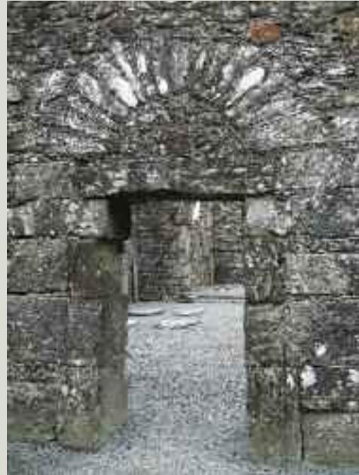
Relieving arch over a flat door lintel
