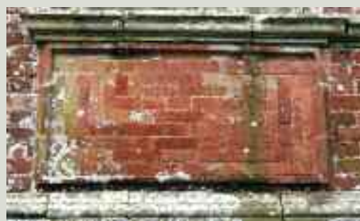
Fine early handmade bricks together with limestone dressings were used in the construction of Palace Anne, County Cork built in 1714
