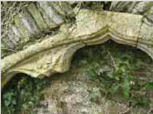
Dundry stone, a cream-coloured oolitic limestone, was popular with mediaeval builders because it could be easily carved. It was imported from Somerset for use in the decorative features of many castles and ecclesiastical buildings
