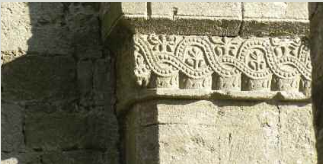
In strong sunlight the marks from the original mason's tools are clearly visible on the surface of the stone (Image courtesy of the Office of Public Works)
