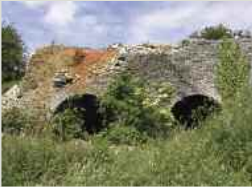
Limekilns were once a common feature throughout the countryside, burning limestone to provide quicklime for use in building mortars or as a fertiliser
