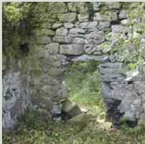
The stones that formed the jambs to this doorway have become dislodged because of cattle pushing through the narrow opening
