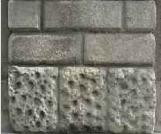
Granite ashlar with vermiculation to the lower course
