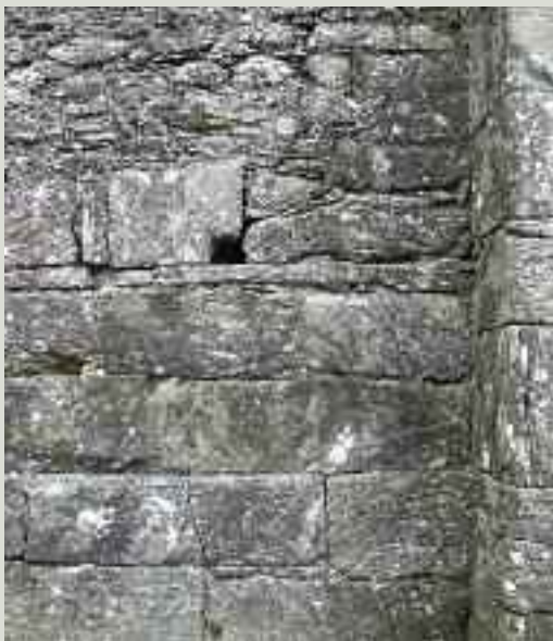
Large blocks of cyclopean masonry can be seen to the lower courses of this wall
