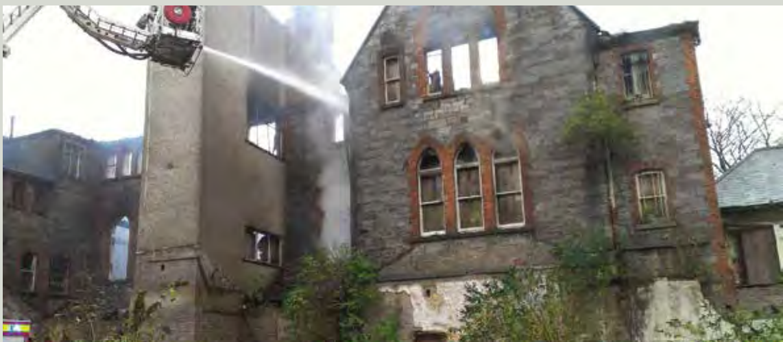
Fire damage is frequently accompanied by water damage. A standard firefighting hose can deliver 500 litres or half a tonne per minute. A hydraulic platform such as that shown here can deliver up to 1800 litres (Images courtesy of Cork City Council)
