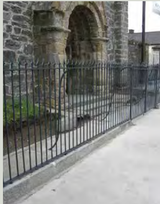
An important twelfth-century Hiberno-Romanesque portal very close to a busy street corner. The risk of impact damage was high as the railings were positioned very close to the doorway, the junction was busy and there was often illegal parking on the footpath. Planning permission was granted to move the railings further out from the building, to widen the footpath and to place bollards to prevent parking on the footpath. The bollards facing the church doorway are removable to allow for funerals
