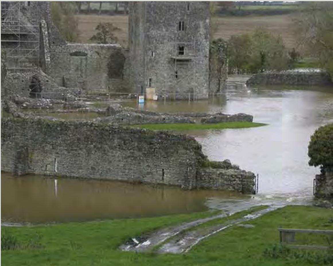
A medieval monastic complex subject to flooding from a nearby river. This type of flooding tends to damage foundations and cause subsidence leading to possible collapse
