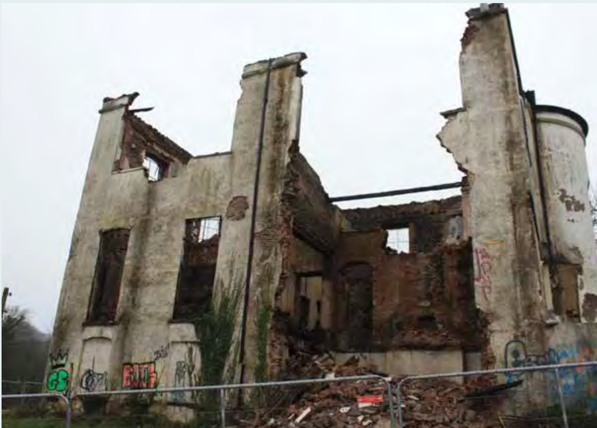
A distinctive eighteenth-century house, unique in its oval plan with curved end-bows, was destroyed by fire. The collapse of a chimney stack during the fire took down the rear wall. It now requires stabilisation to prevent further collapse, pending decisions regarding its future
