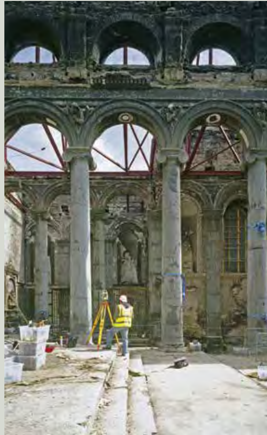
Once the structure has been made safe, a survey of the extent of damage can begin (Images courtesy of ARC Consultants)
