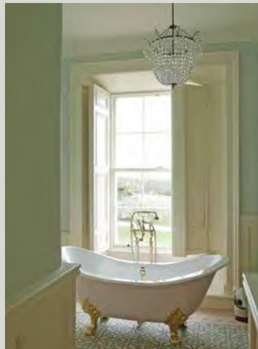
Water damage – before and after repair and redecoration (Images courtesy of ARC Consultants)
