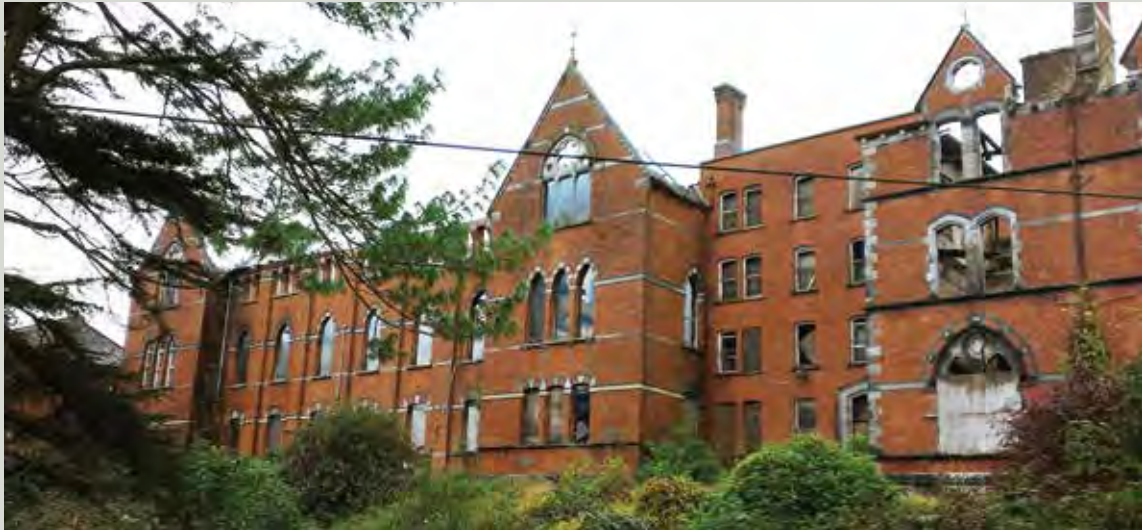
A large building gutted by fire with roof and upper floor levels totally destroyed
