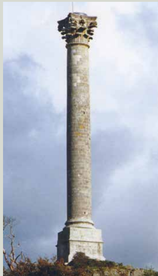
The repaired Browne-Clayton Monument with the newly-fitted lightning conductor just visible at top left of centre (Image courtesy of Rainey's, Swords)
