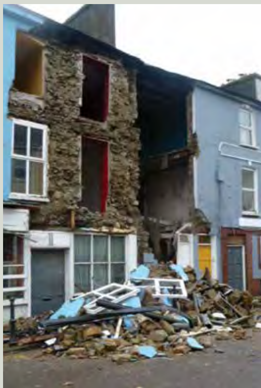
Alterations including the use of inappropriate materials such as cement render on a historic building trap moisture within the structure behind, causing decay and in some cases can lead to catastrophic failure
