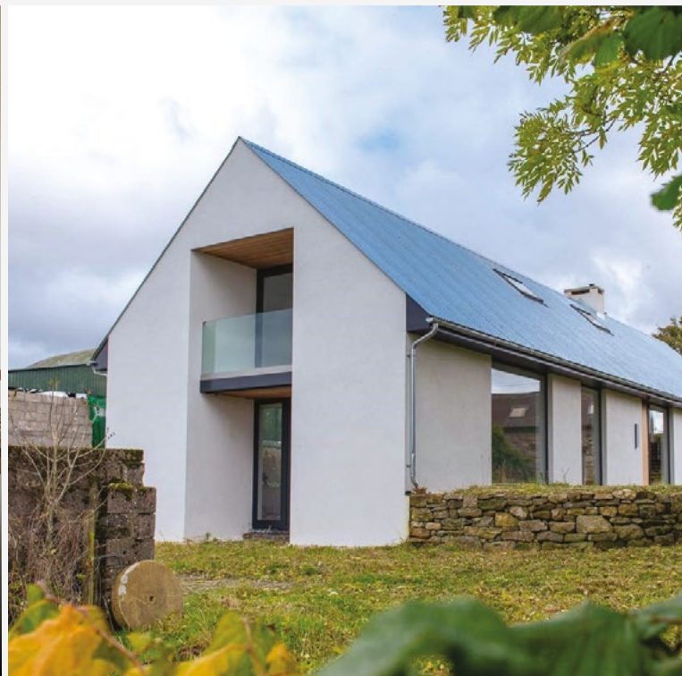
The retention in use of an original farmhouse through the careful insertion of contemporary accommodation respecting the setting and historical character of the original farm complex. Photography: Peter Grogan, Emagine
