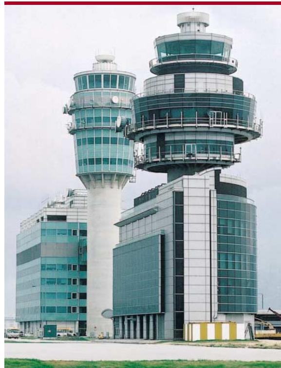
航空交通管制大樓(左)和作備用的大樓(右)。備用大樓頂部裝有精密跑道監察系統。 Air Traffic Control Complex (left) and the one used for backup purpose (right). The Precision Runway Monitor was installed at the top of the backup complex.
