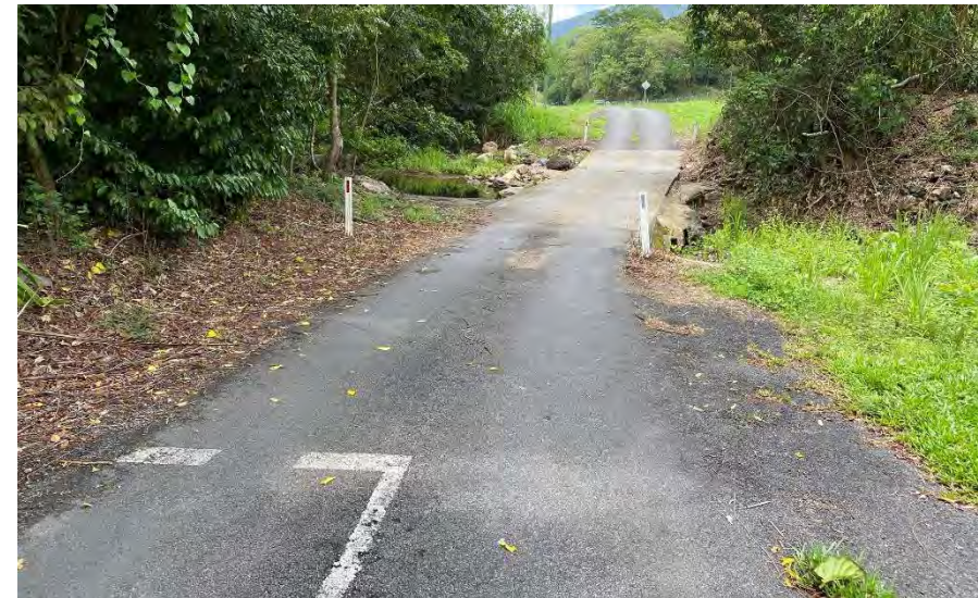
Bottom Right: Waterway crossing (Brays Road, Little Mulgrave)
