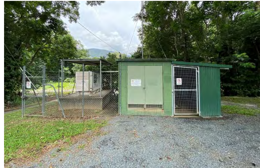
Top Right: Water Treatment Plant (Papacek Access, Little Mulgrave)
