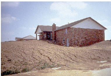
US Environmental Protection Agency Poorly graded slope (Slopes should be roughly graded to slow runoff velocity.)
