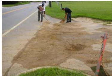
R. Schnabel, Chesapeake Bay Foundation Dirt tracked onto adjoining roads by heavy equipment
