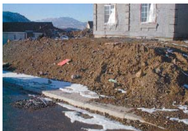
US Environmental Protection Agency Unprotected slope (Immediately after construction, slopes must be seeded and covered with mulch or geotextile material.)
