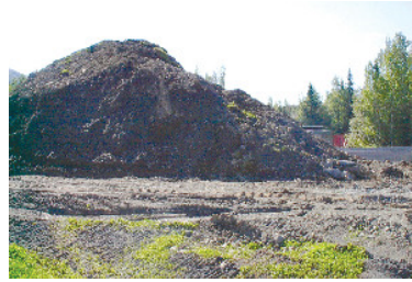
US Environmental Protection Agency Uncovered dirt pile (Dirt piles should be temporarily seeded to prevent erosion.)
