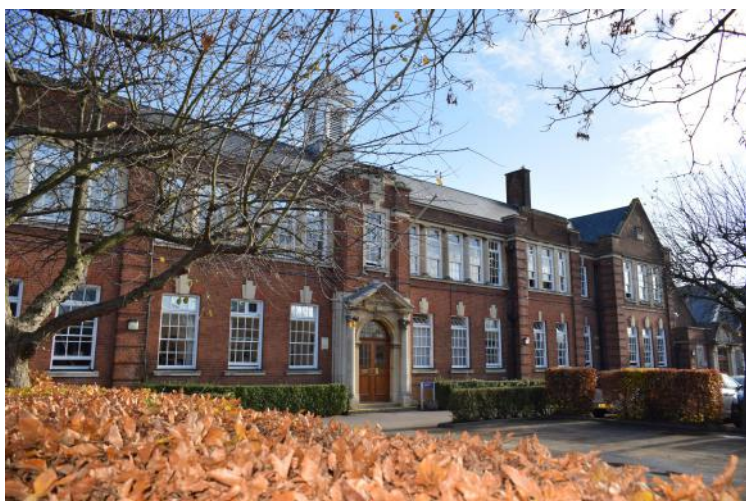
Photo of the school taken in November 2020 after replacement of the roof tiles.
