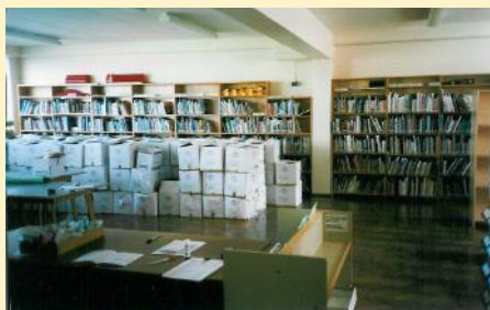
Photos taken during the Library refurbishment in 1999. Students were obviously helping out with the removal and storage of books during the work.
