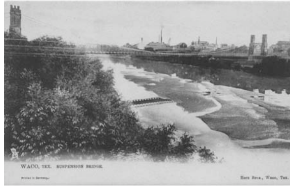
Figure 3. Waco Bridge (David Denenberg collection)
