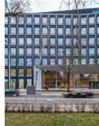
Project Green2Day Location Wroclaw, Poland GLA 17,000 sqm Completed Q4 2017 Developer Skanska Commercial Development Europe
