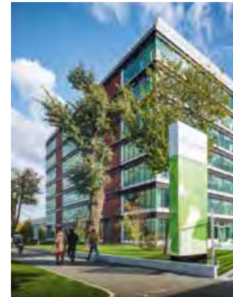
Project Oregon Park - Building B Location Bucharest, Romania GLA 24,000 sqm Completed Q1 2017 Developer Portland Trust
