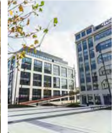
Project Mechanica 1&2 Location Prague, Czech Republic GLA 32,000 sqm Completed Q3 2017 Developer Penta Real Estate
