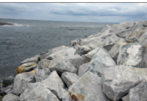
New rock revetment wall. Michael Brubaker 2010.
