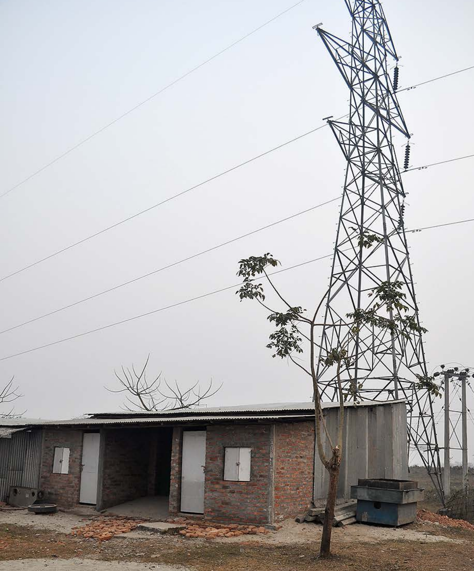
Government of India transmission lines pass above a town with a DESI Power microgrid in Bihar, India.
