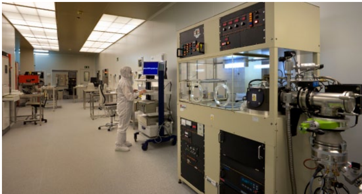
Integrated Micro and Nanoelectronics Clean Room and associated laboratories for microsystem processing, encapsulation and electrical characterization at the Instituto de Microelectrónica in Barcelona. The Spanish Ministry for Economy and Competitiveness classifies it as a Special Scientific Facility.
