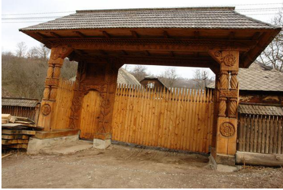
Wood gate in Maramures
