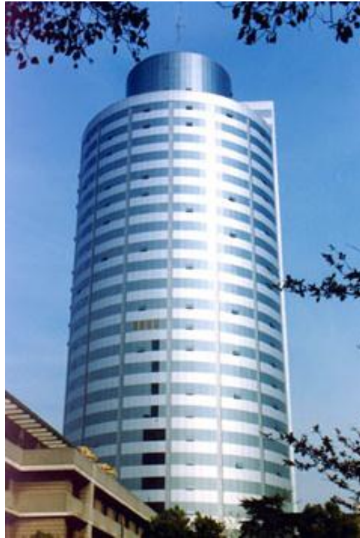
Fig. 4.108 – Building with curtain walls
