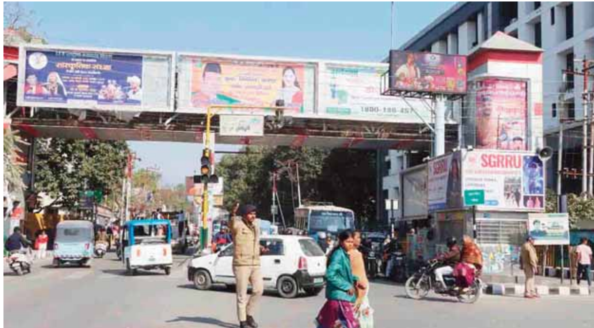
The pedestrian overbridge at Tehsil Chowk in Dehradun, inaugurated in 2015 remains locked after considerable expenses as pedestrians walk across the road and the structure remains a base for advertisements Mangesh Kumar/Pioneer photo
