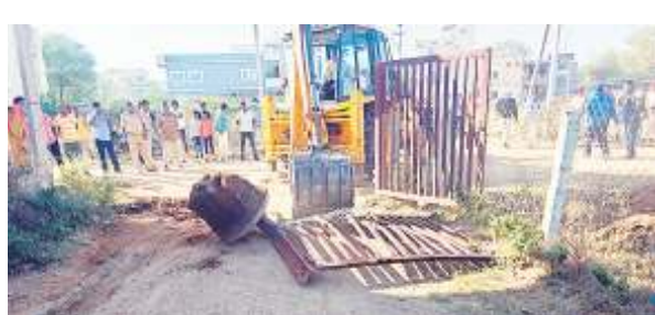
The demolitions of illegal constructions by HYDRAA in Shamshabad
