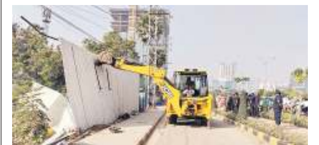
HYDRAA demolishing illegal structures near Khajaguda-Nanakramguda main road in Serilingampally mandal
