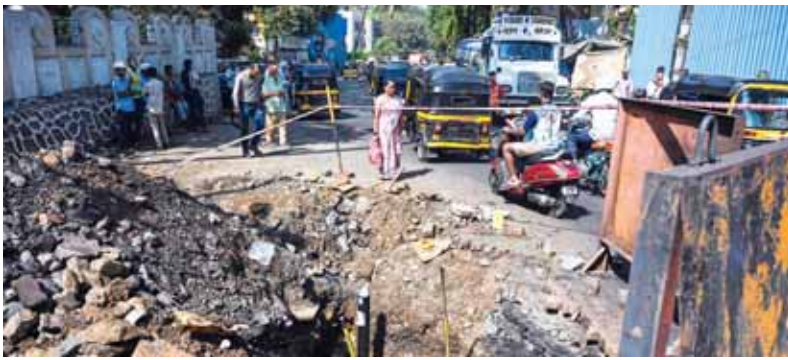
Repair work underway after leaking of a gas pipeline in Mumbai
