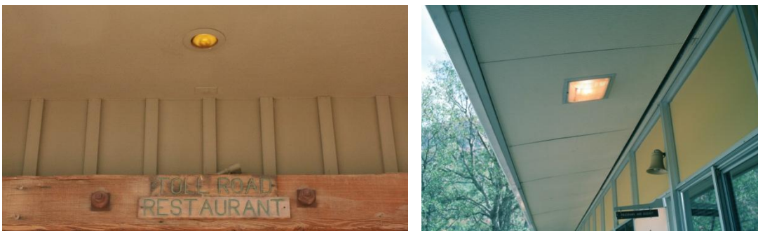
Figure 14 a-b. Recessed under canopy lights at Stovepipe Wells (left) and Sequoia National Park (right).
