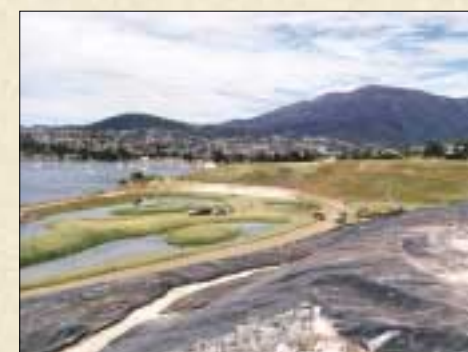
Pasmenco landfill rehabilitation
