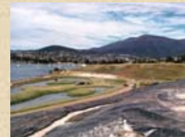
Pasmenco landfill rehabilitation
