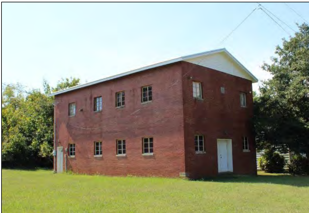
Charlotte Lodge No. 146, Wilson Street, northeast oblique, 2021.
