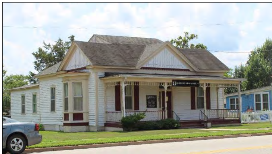
191 King Street, northeast oblique, 2021.
