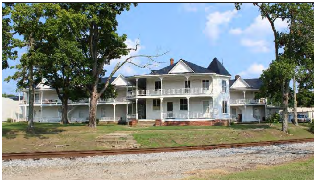
Hotel Charlotte, west elevation, railroad tracks in the foreground, 2021.
