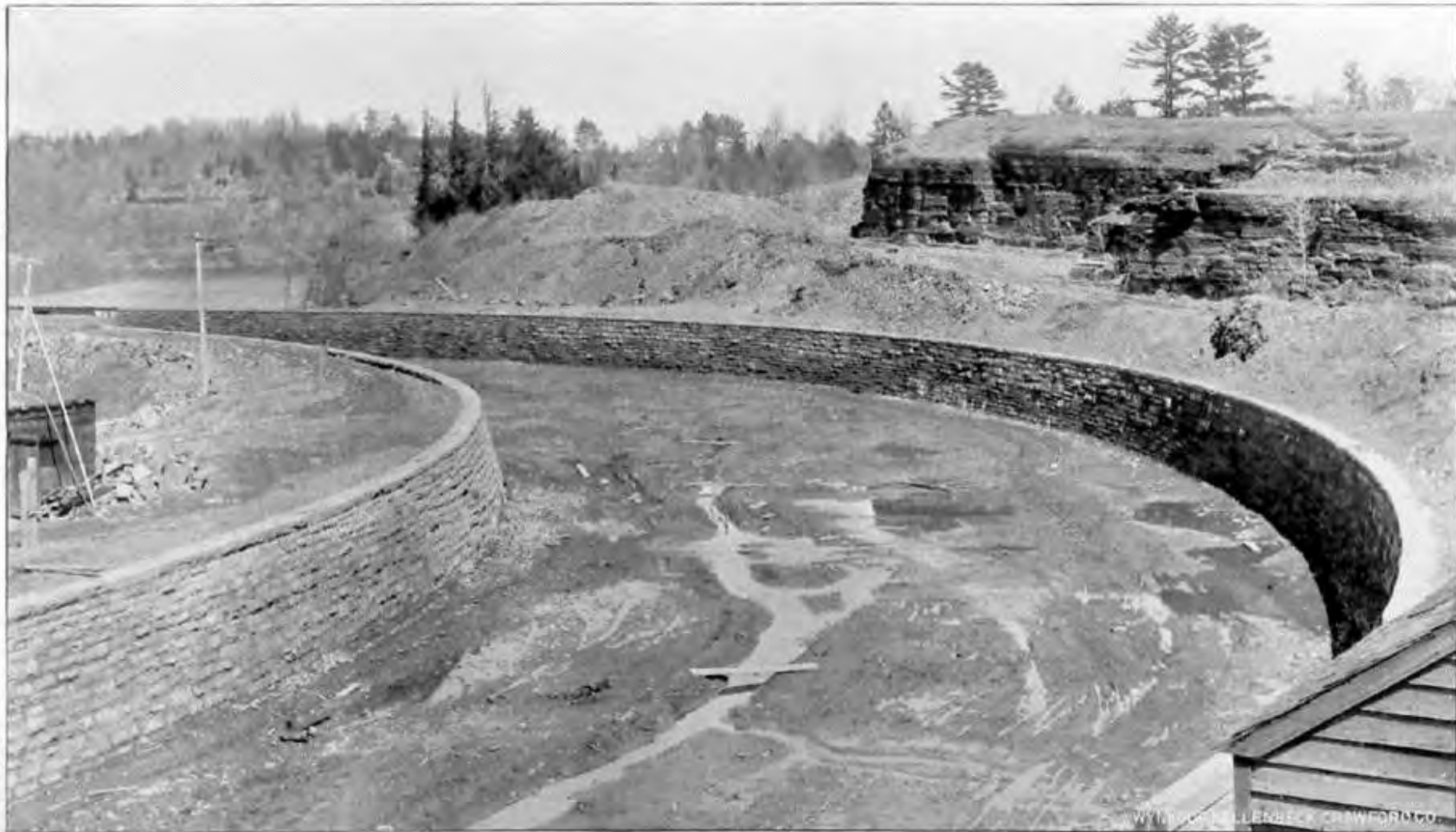
NEW VERTICAL WALL AT ENTRANCE TO UPPER MOHAWK AQUEDUCT.
