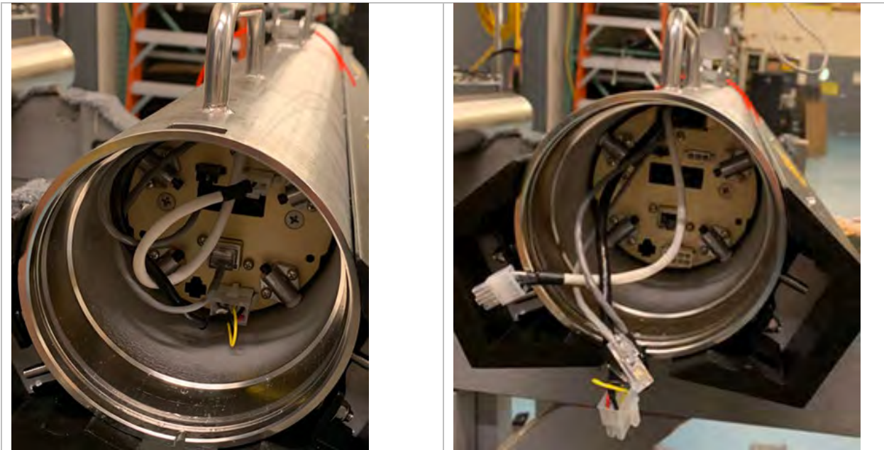
Figure 7-6: Forward Endcap Cable Disconnections
