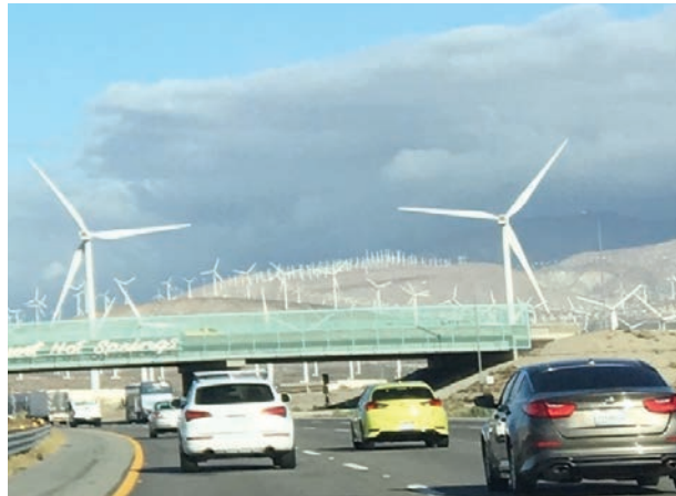
Wind turbines near the San Geronio Pass
