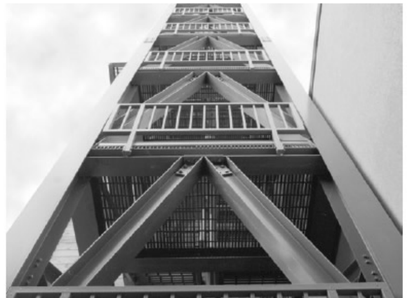
A 63' (19.2m) high freestanding fiberglass stair tower at Ft. Story Army Base, Virginia Beach, Virginia.
