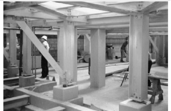
EXTREN® structural shapes were used in a SXEW copper refinery because of the highly corrosive environment.
