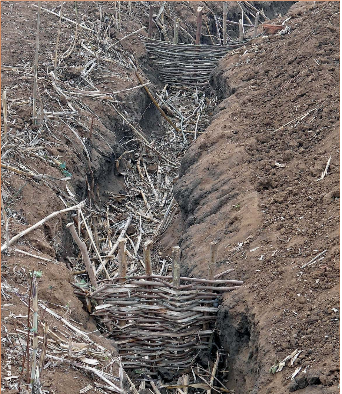
Figure 27: Sediment trapping in a gully. Zomba, Malawi.
