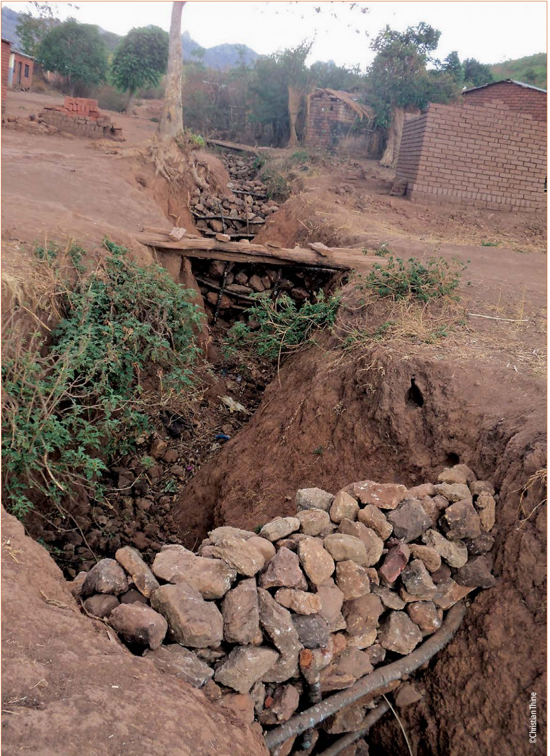
Figure 29: Check dams used to halt gully erosion in to a village. Ncheu, Malawi.
