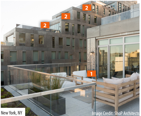
New York, NY Image Credit: ShoP Architects 1 Residential balconies provide relief to building form and create extensions of habitable spaces 2 Multiple step-backs create a downward transition in height through a series of terraces
