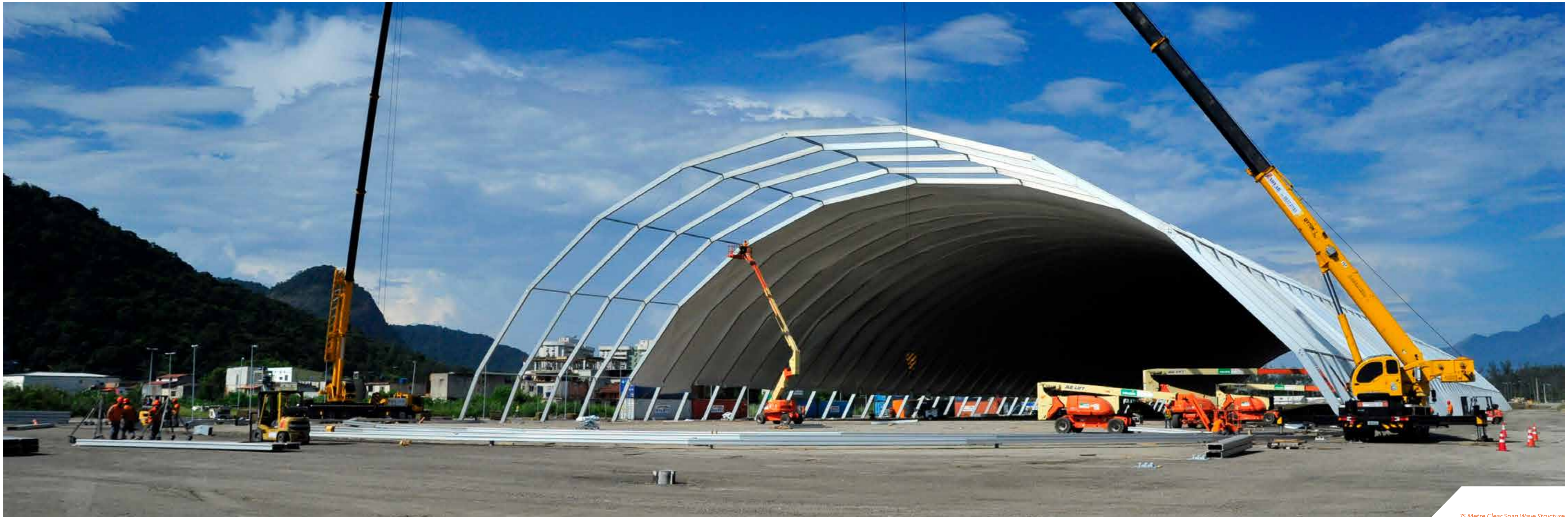
75 Metre Clear Span Wave Structure
